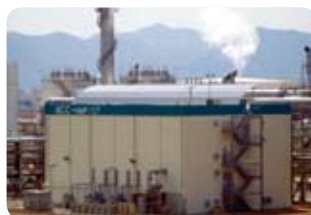
GS Caltex Factory(50kW)
