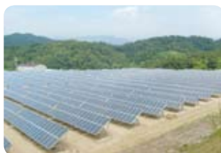
Young Ju PV Plant(1MW)
