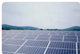
Young Gwang PV Plant(2.5MW)
