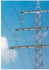
110kV Line (Germany)
