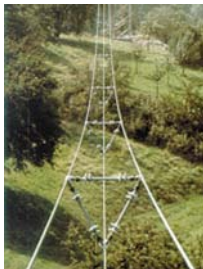
20kV Line (Germany)
