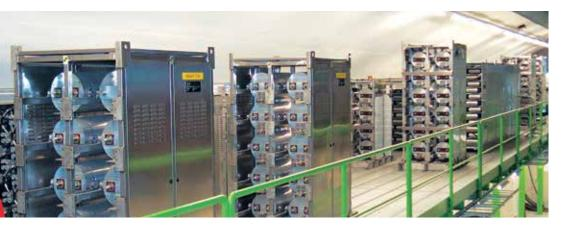
Braking Resistors for large motors are customised to best comply with any requirement: we have developed special Braking Resistors for important research institutes (among them Max Planck Institute) and for energies in excess of 3400MJ.
